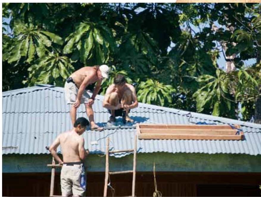
Future Scientist members Tyson Kim, Bob Pollard, and Richard Novak install solar panel framing on the roof of the orphanage director's house. The panels now power a laptop and TV and reduce usage of a gas-powered generator.
